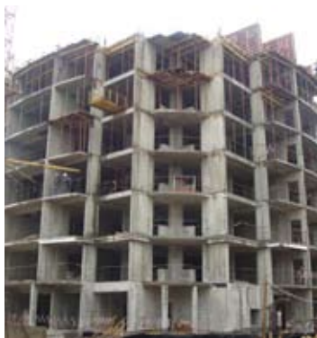
Emerald Valley Residential Complex
